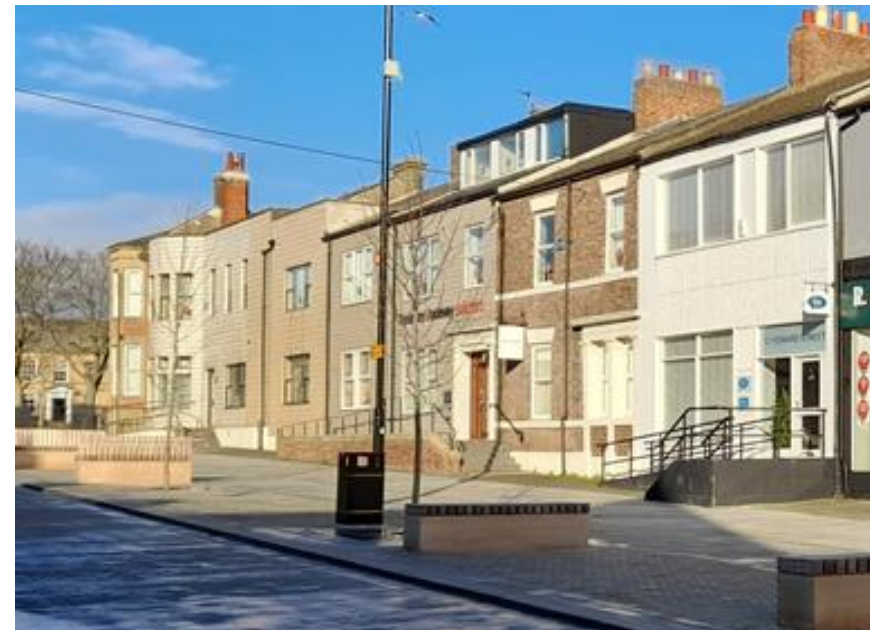
Tiled properties at the northern end of Howard Street
