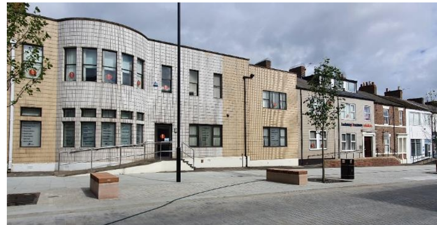
Inappropriate materials on Howard Street
